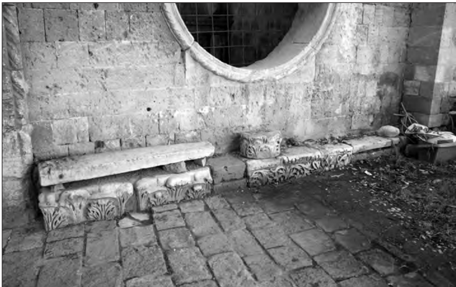
Figure 6. Classical Entablatures and Capitals from Salamis Used to Continue the Panca or Bench along the North Side of the Loggia Bembo in Famagusta's Main Square – Allan Langdale
